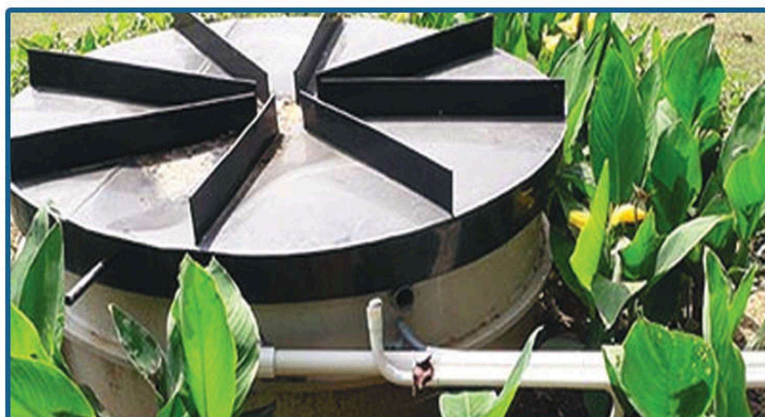
SEWAGE TREATMENT PLANT
