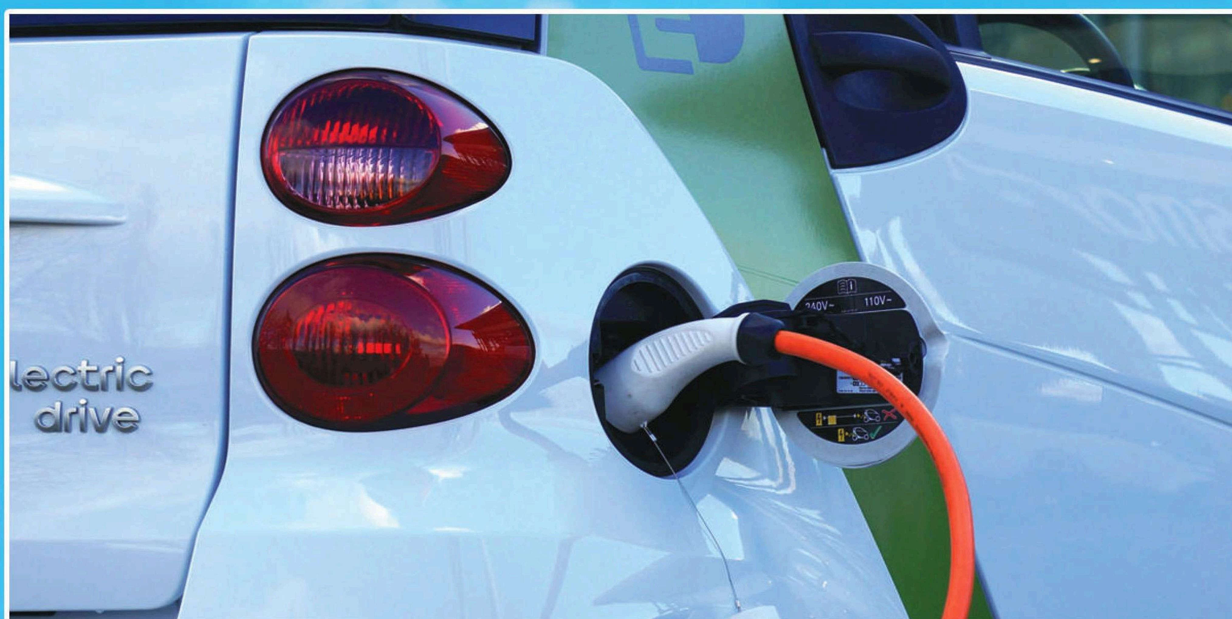
E-VEHICLE CHARGING STATION
